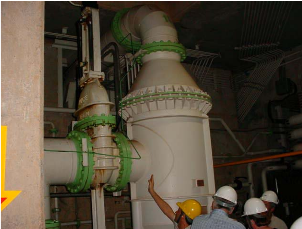
Figure 4: Service water filter. Inlet from above, outlet on left side.
