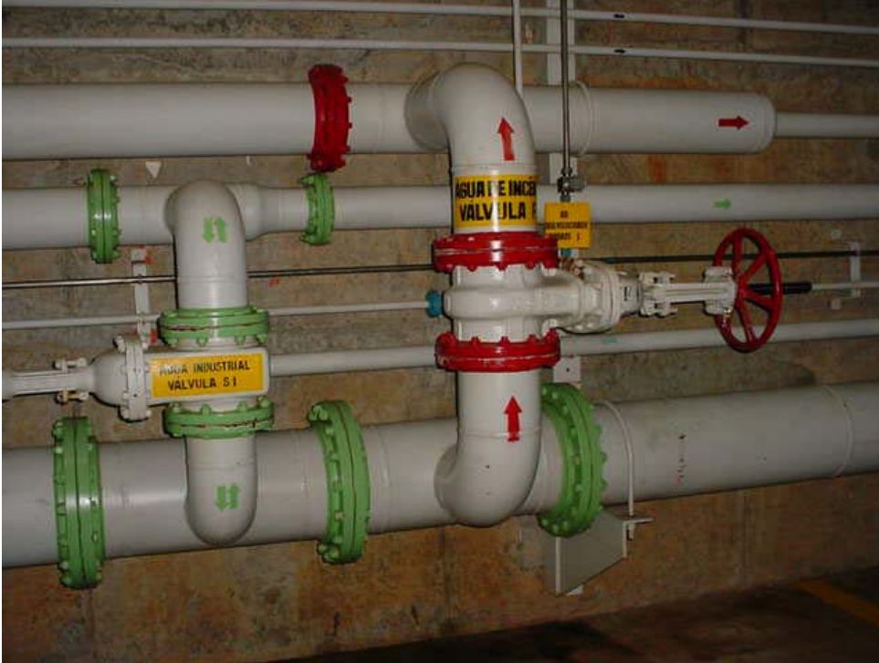
Figure 5: Fire water take-off (red piping) from service water common header (green piping)
