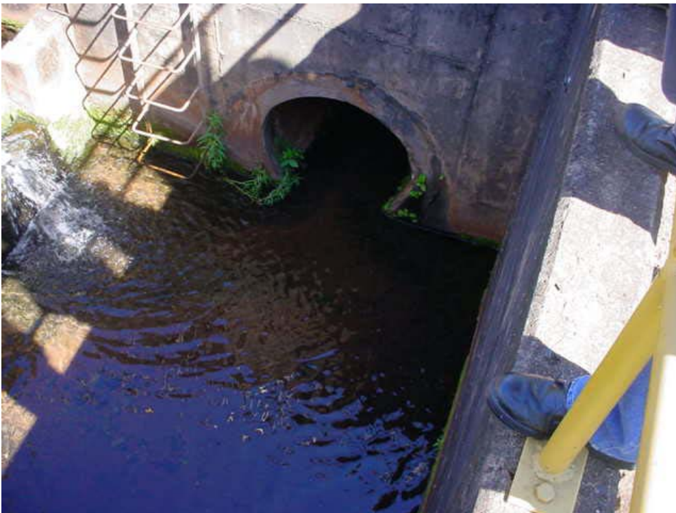
Figure 6: Drain piping from toe of dam.
