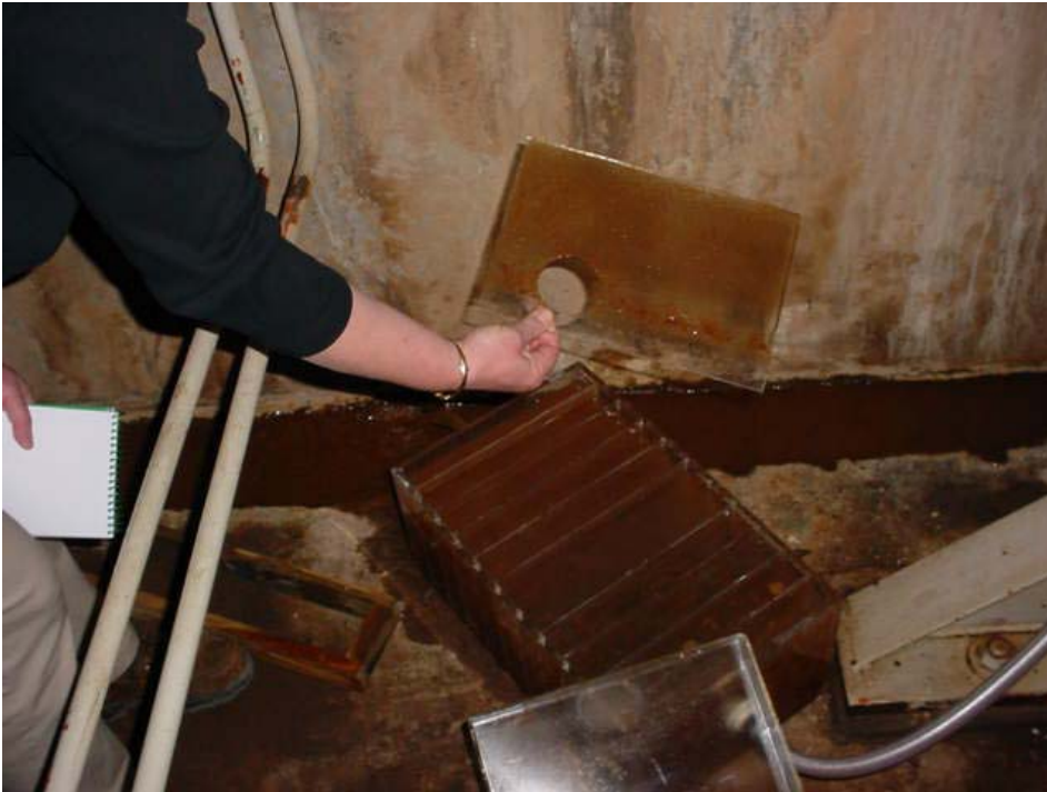
Figure 3: Bio-box at service water take-off. There is one bio-box for each of the 6 units.
