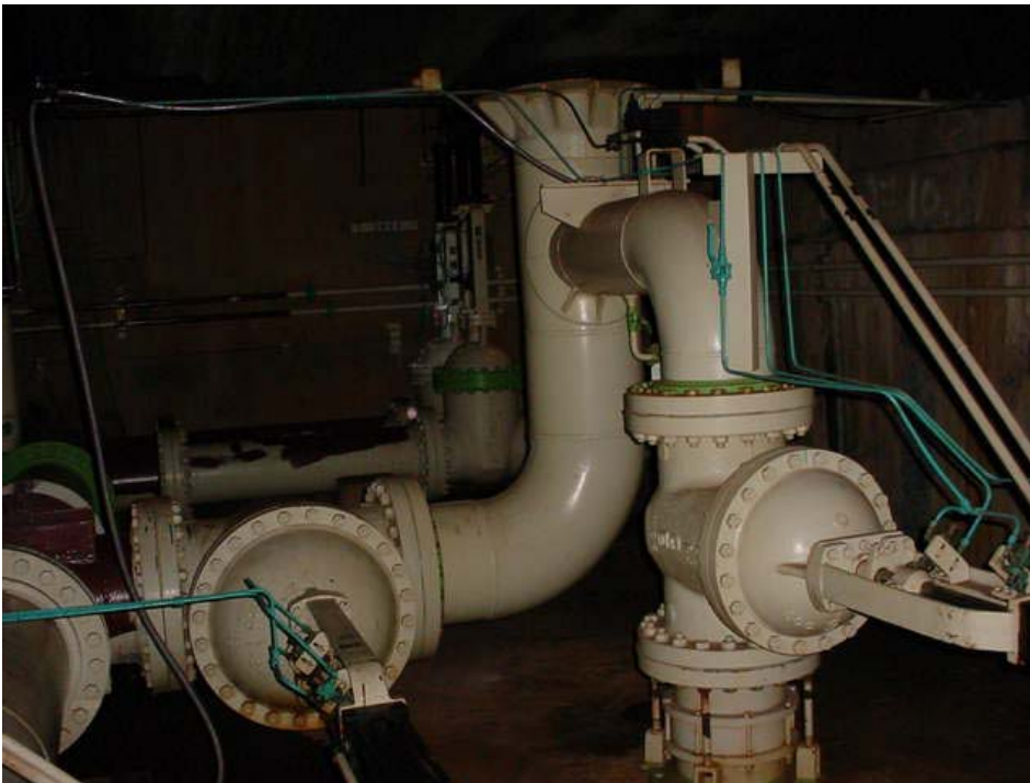
Figure 2: Service water take-off from penstock (penstock is large black pipe at top of photo)
