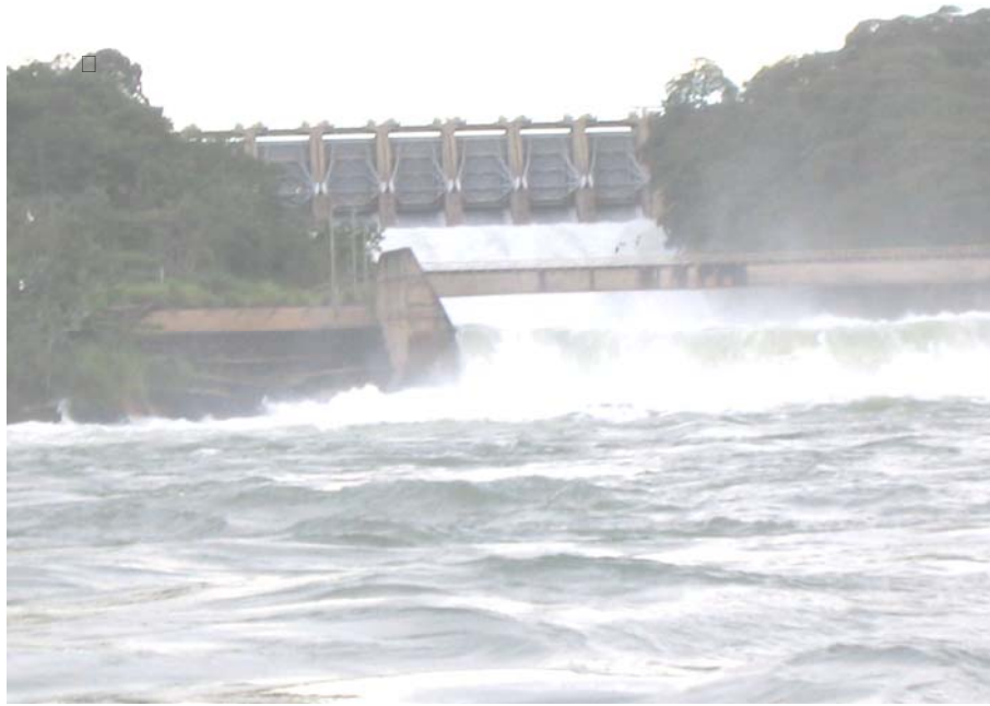
□ Image 1. Reservoir overflow. Note the extreme turbulence as the reservoir water meets the river at the base of the spillway.
