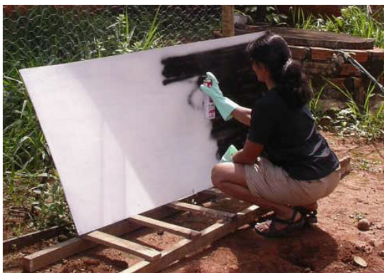
5. Painting metal floor black to absorb heat
