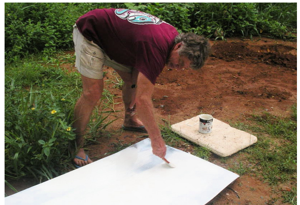
4. Painting primer on metal floor of solar chamber
