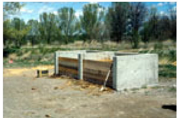
12. Bins for composting fish mortalities in a 2-stage system at Buhl, Idaho.
